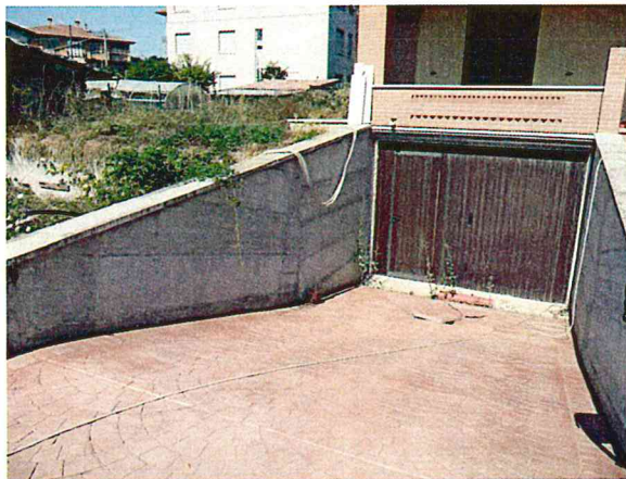
Foto 8 = rampa garage (lotto 1)
